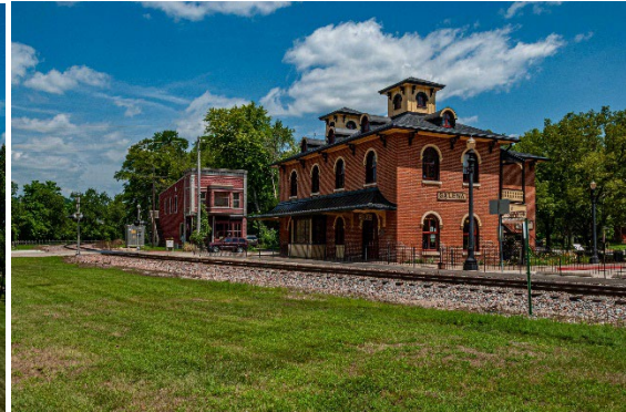
Illinois Central Railroad station – Galena, Illinois
