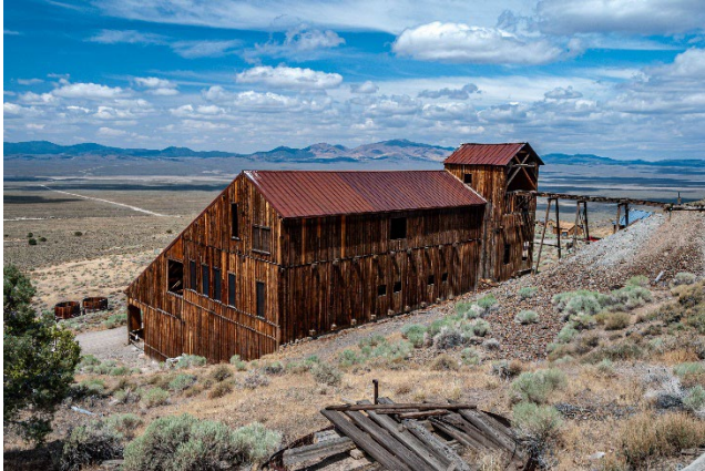
Ore processing building – Berlin, Nevada
