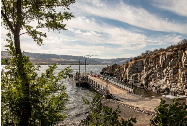
Keller Ferry landing
