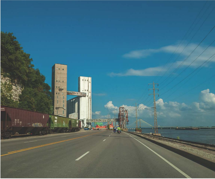
Grain Elevators at Alton, Illinois
